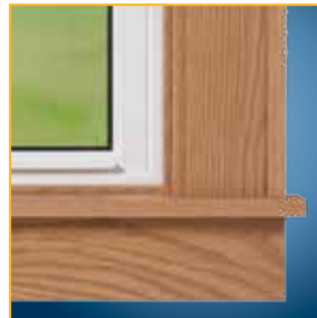
FLAT WITH BACKBAND IN STOOL AND APRON
