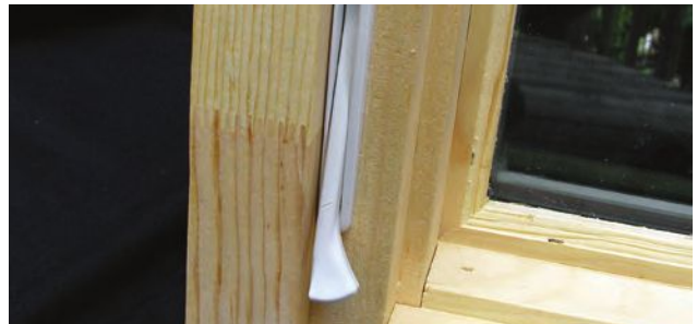
Encore Multi-Point Locking System A fully concealed locking system. White hardware standard. Bronze is optional.
